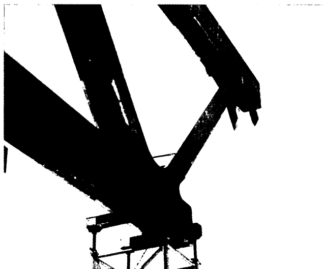
Figura 18. Barras y nudos de Puente sobre el río Sil, durante el ensamblaje en obra/ Figure 18. Members and joints to the bridge over the River Sil during assembly on site.
