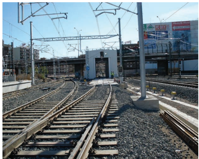
Foto 12. Cambiador de Ancho de Valencia. Lado ancho. The image shows a railway switch structure from a different perspective, showing the tracks curving through the structure. The structure is white and modern, situated in an open area with tracks and overhead power lines visible.
