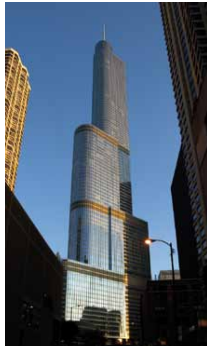
Trump International Hotel & Tower, Chicago (2009, 423,22 m)
