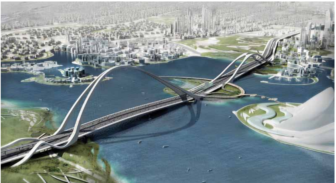
Fig. 26. Sheikh Rashid bin Saeed Crossing
