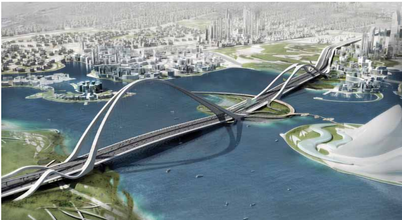
Fig. 26. Sheikh Rashid bin Saeed Crossing
