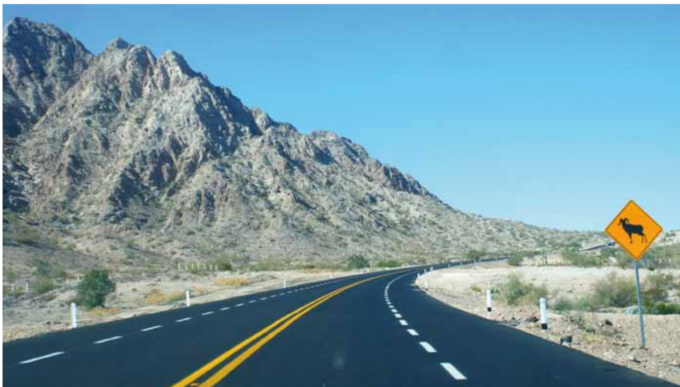
Carretera Sonoyta-San Luis Colorado (Comsa Emte)
