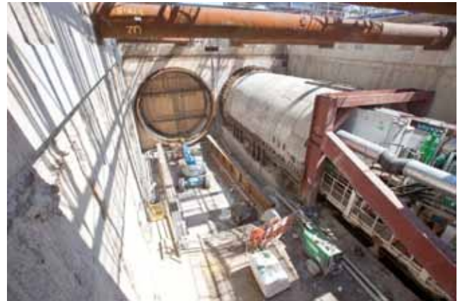
Fig. 2. Royal Oak portal. Main tunnel site
