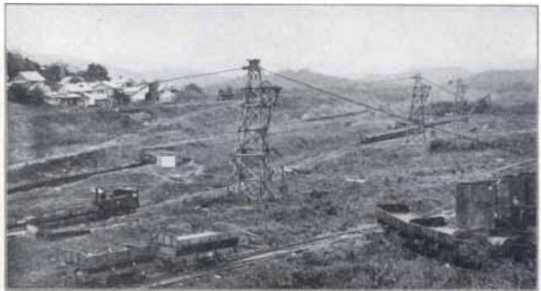
The Cut in French times, showing their cableway plan of excavation. These cableways carried the material out of the canal and deposited it to one side, but unfortunately not far enough, for much of it has slid back into the Cut, causing extra excavation.
