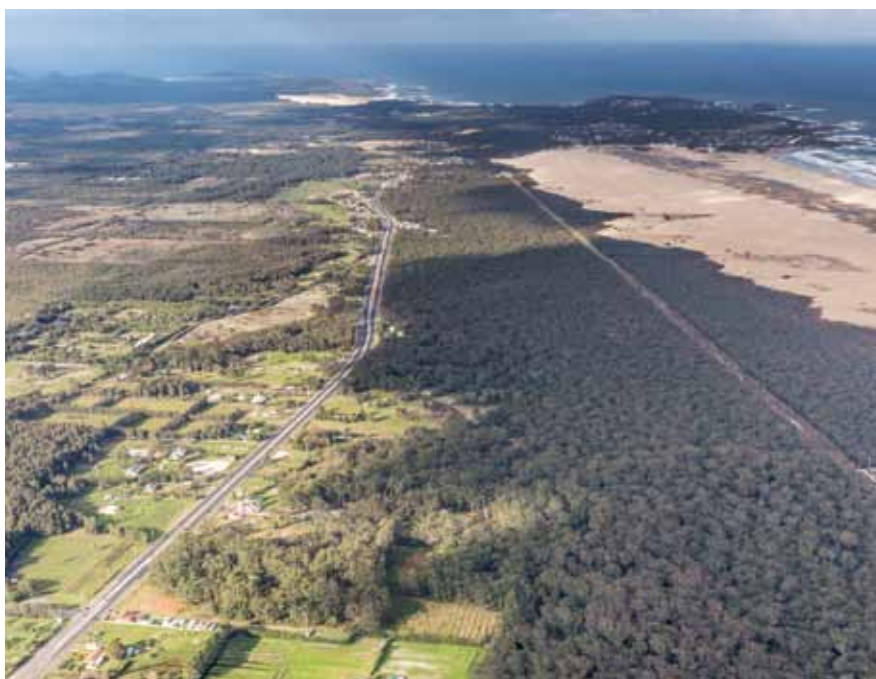
Nelson Bay Road (Ferrovial)
